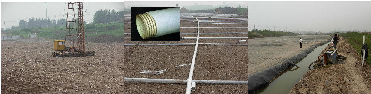
Fig 1. Site layout of vacuum preloading (a site in Nanjing, China)
